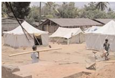
Tents and wooden shelters under construction in Moratuwa
